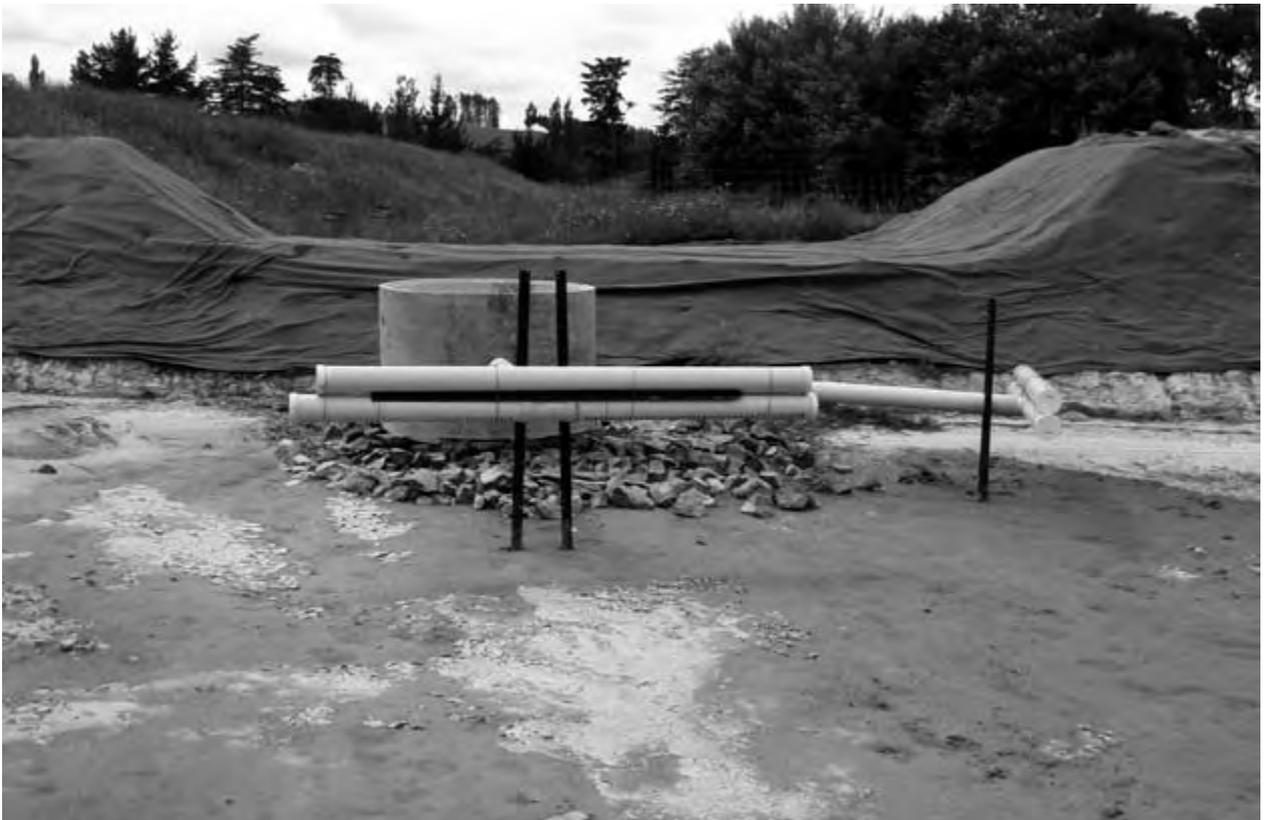
**Plate 12: Sediment retention pond showing decant system.**
