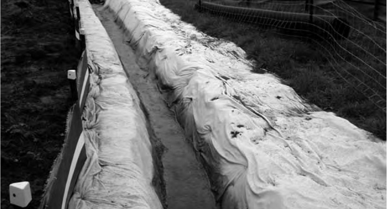
**Plate 1: Runoff Diversion Channel**
