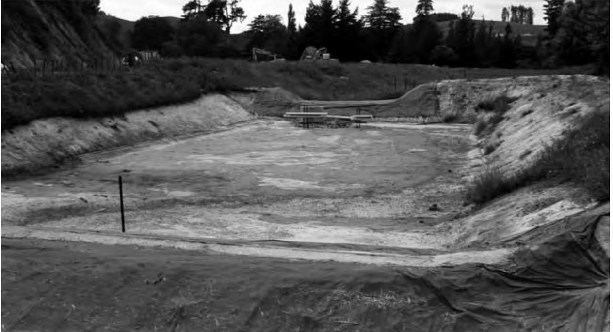
**Plate 11: Sediment retention pond showing decant systems**
