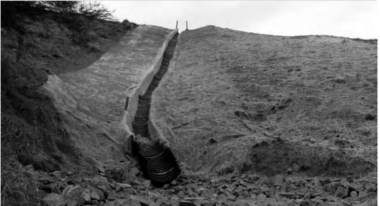
**Plate 9: Flume drop structure**
