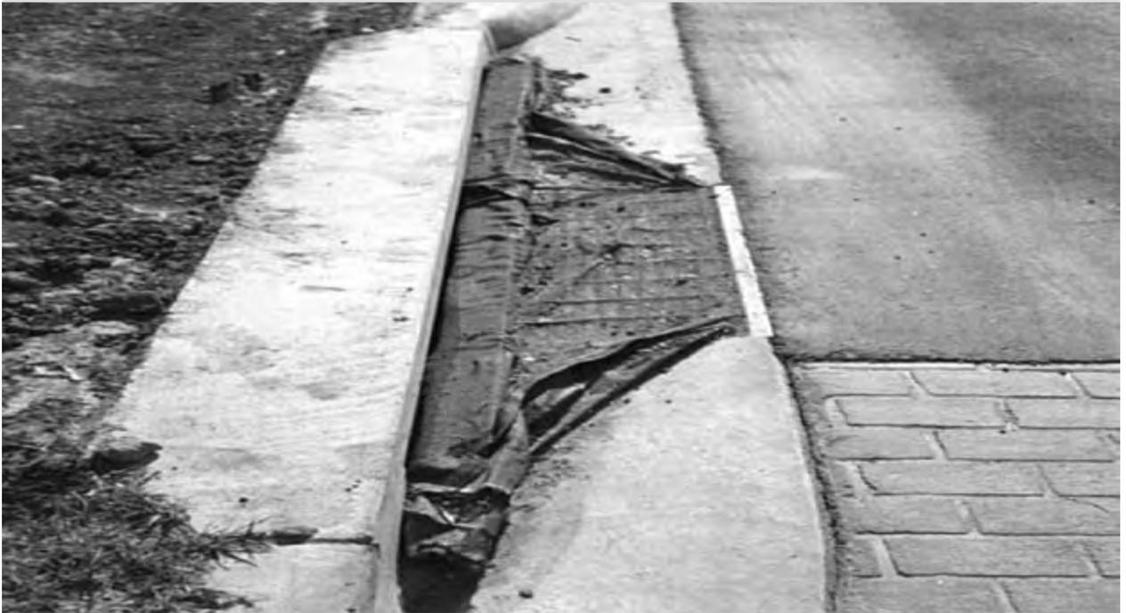
**Plate 16: Stormwater inlet protection**
