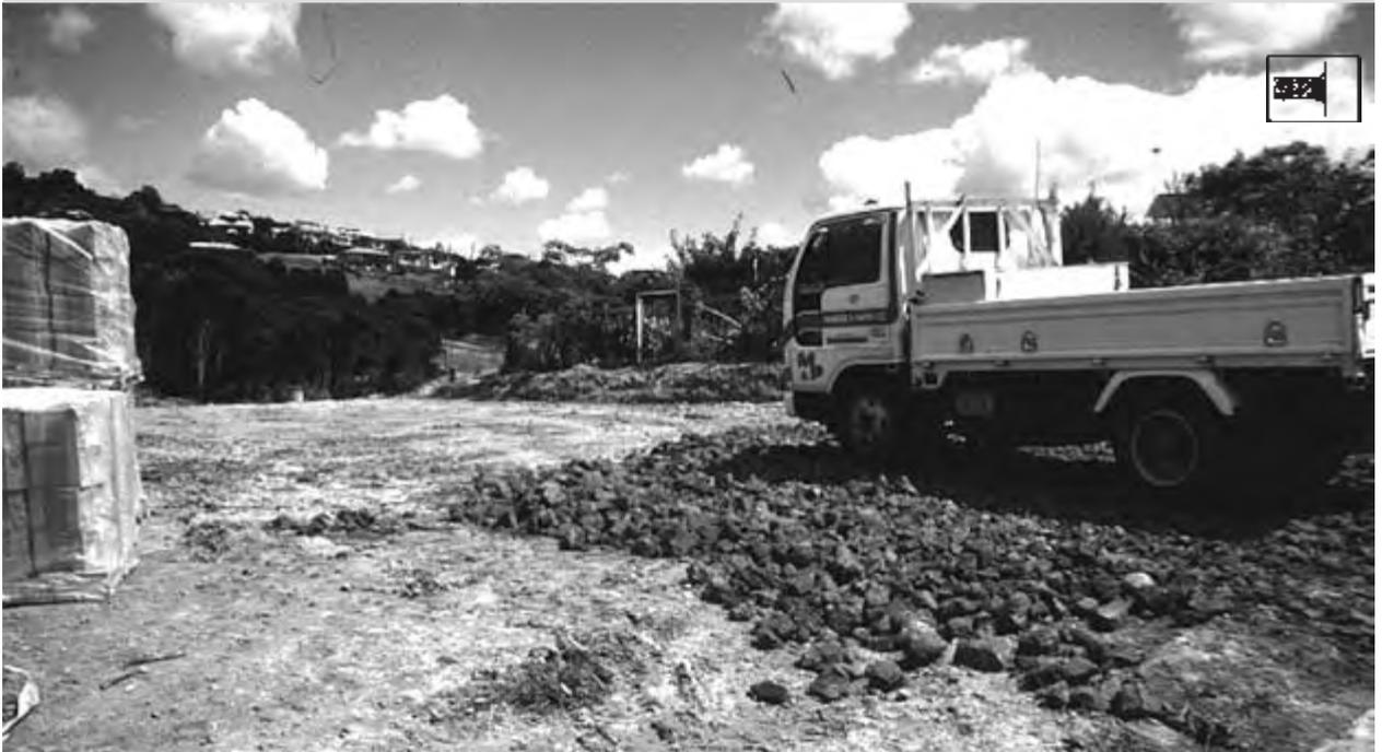
**Plate 8: Stabilised Construction Entrance**
