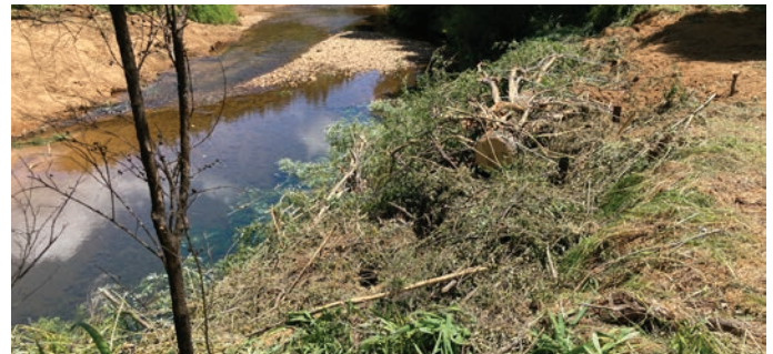
Tree layering along the Kaimarama River helps protect the bank from erosion.
