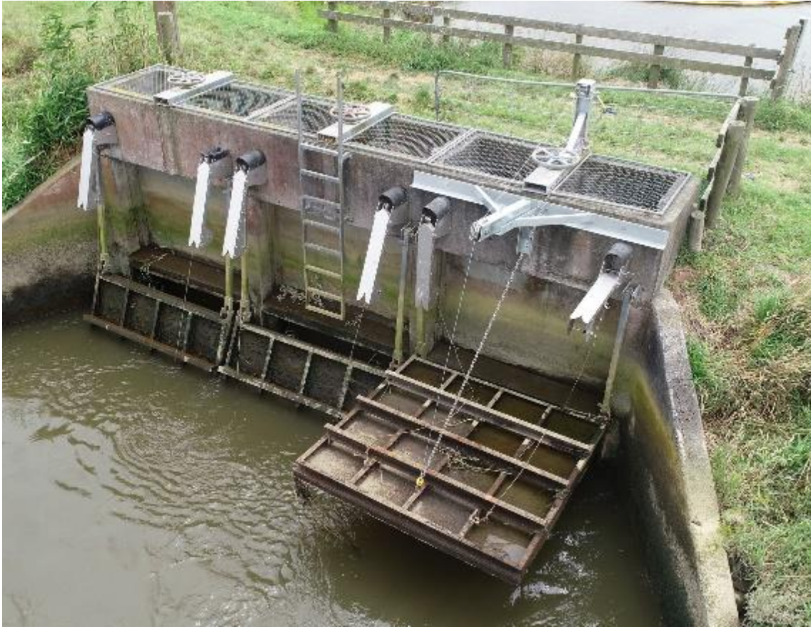
Figure 26: Aka Aka floodgates when the winch was installed
