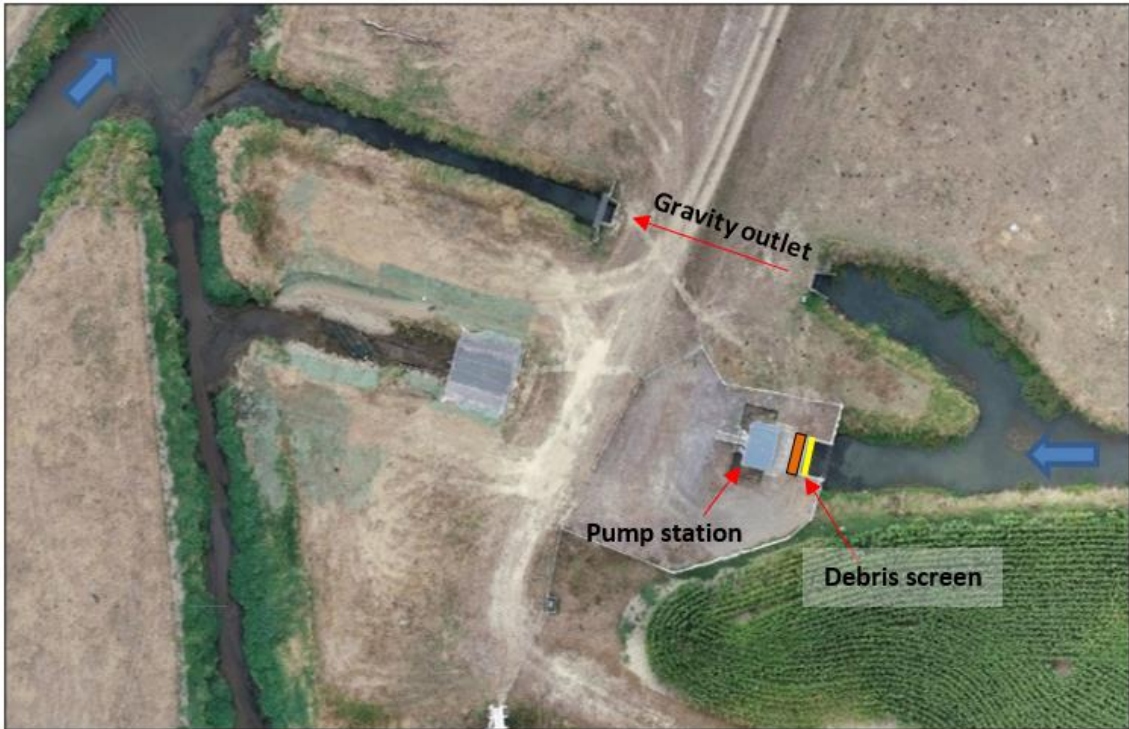
Figure 9: Aerial view of the Steiners pump station showing the two outlets and the direction of water flow (blue arrows). The experimental electric barrier system (orange rectangle) was installed behind the debris screen (yellow line)
