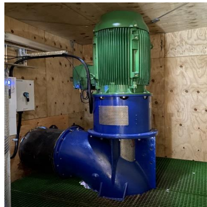
Pump installed at Huntly Golf Course pump station
