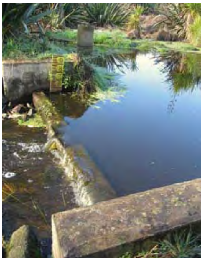
Minimum water levels help protect the lakes by reducing the impacts of drainage immediately downstream. This weir is installed at Lake Koromatua.
