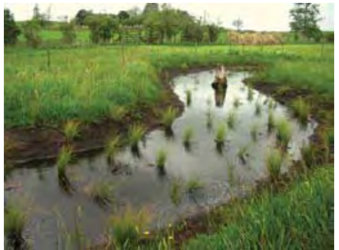
Silt traps have been constructed on all drains entering Lake Kainui. Once the native plants have established, the trap will have similar functions – and benefits – to a wetland.
