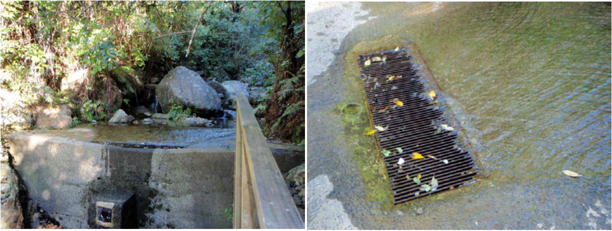
Plates 13 and 14: Weir and water intake for the Te Aroha potable water supply at the downstream end of monitoring locality WS8.
