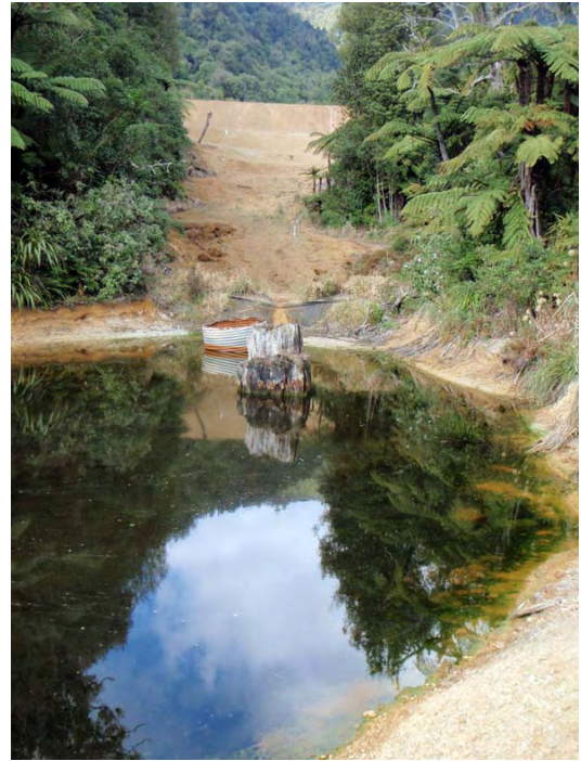
Plate 2: Stormwater / leachate pond for drainage from the Tui Mine Tailings Dam that drains into the Tui Stream.
