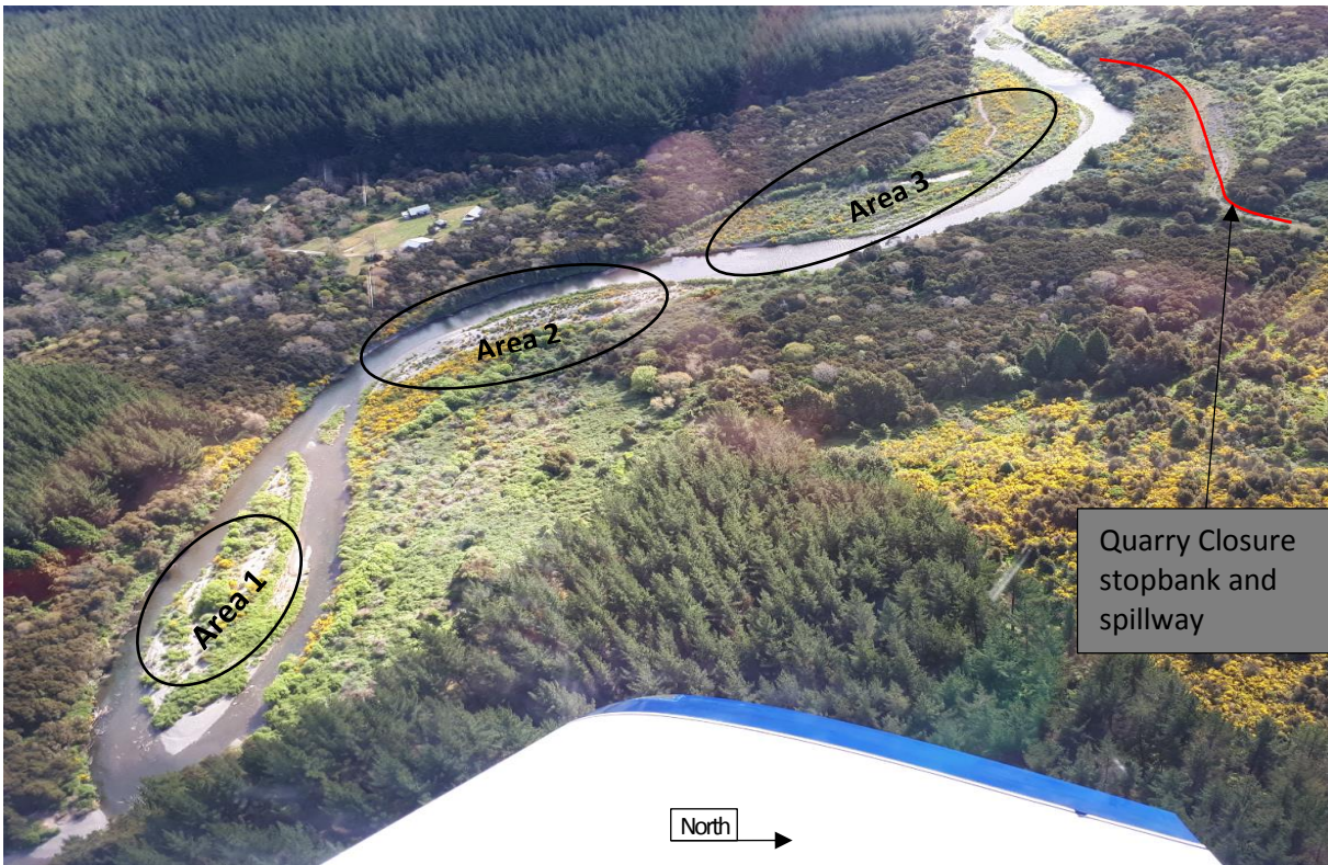
Quarry Closure Stopbank Oblique aerial photo 14 November 2017
