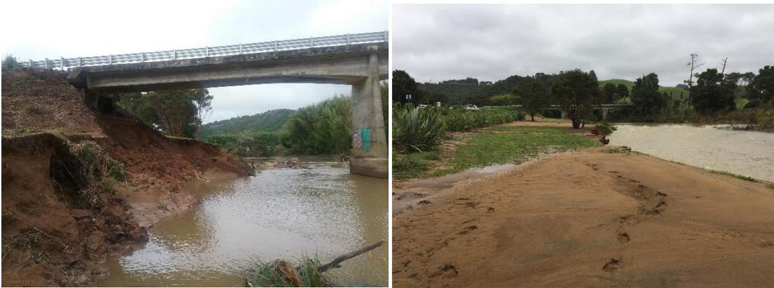
**Figure 13: Photographs taken on Thursday 9 March showing erosion under the State Highway 25 Bridge over the Waiwawa River (left), with silt deposits showing the extent of inundation (right).**
