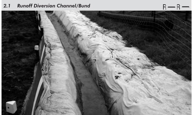
Plate 1: Runoff Diversion Channel
