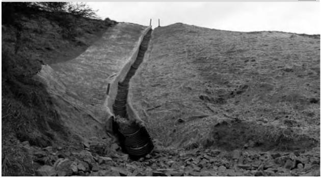
Plate 9: Flume drop structure
