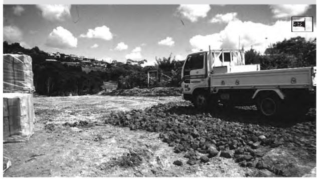
Plate 8: Stabilised Construction Entrance
