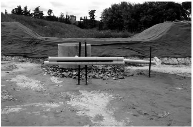
Plate 12: Sediment retention pond showing decant system.
