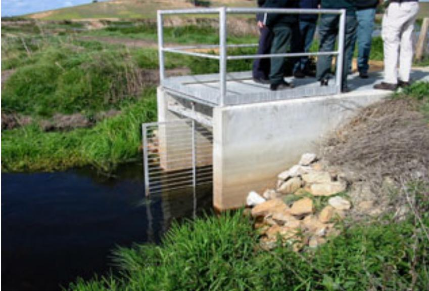
**Figure 32: Flow controller, water inlet and barrier for carp trap - McLeod Morass**
