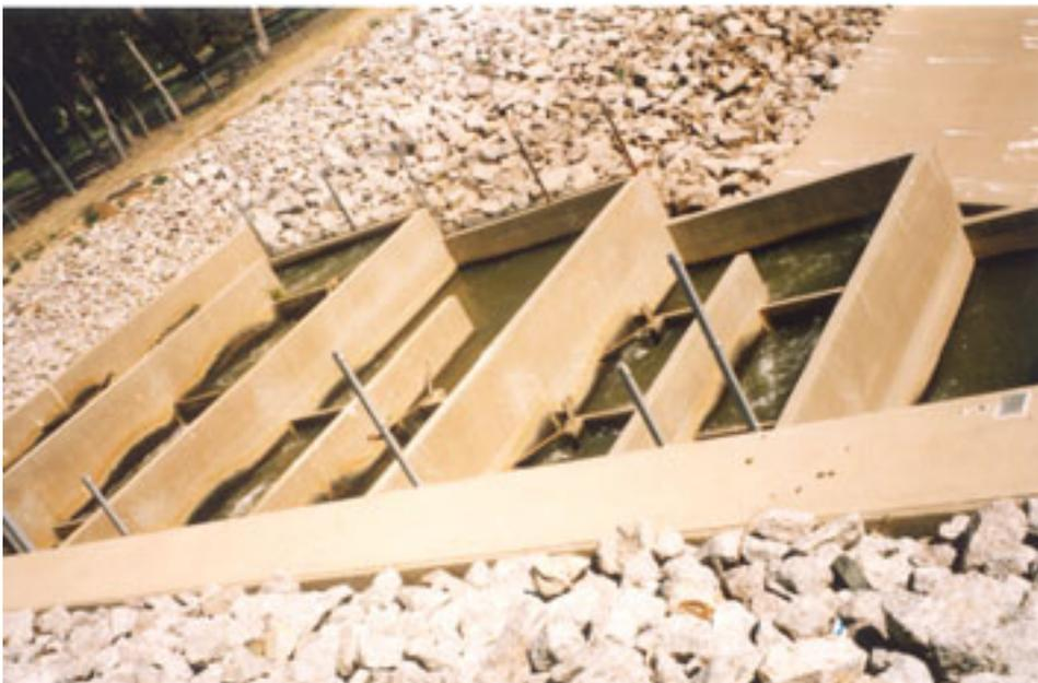
**Figure 3: Fish pass on Torrumbarry Weir**
