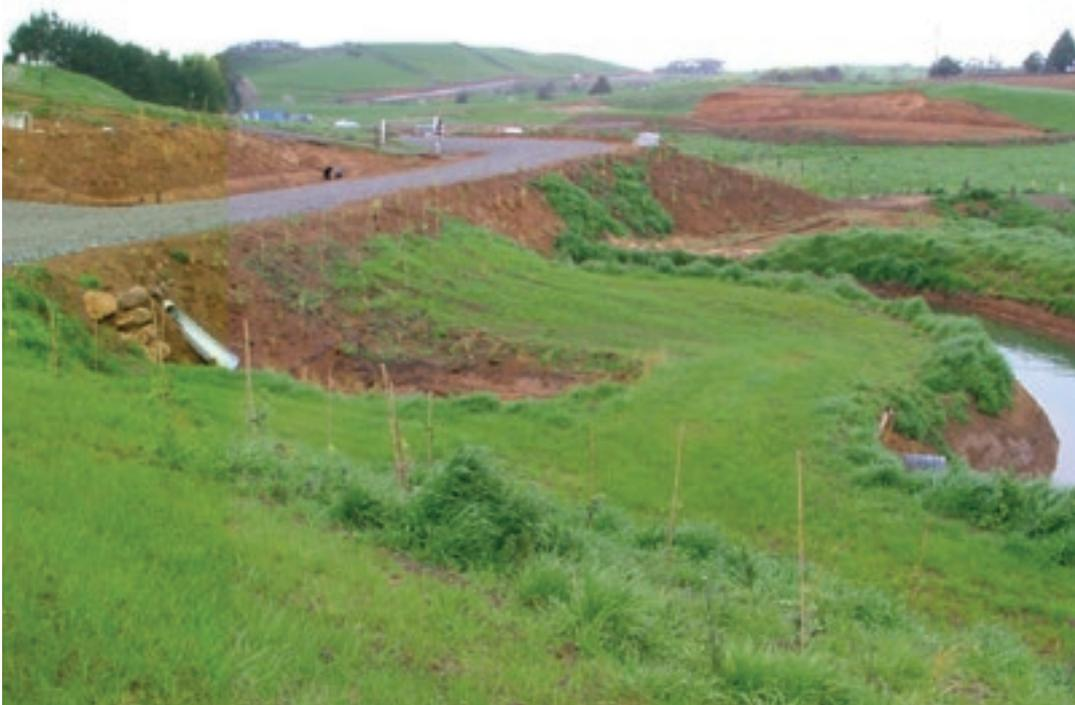
Recently completed earthworks. Note the site has been revegetated to stabilise against erosion.
