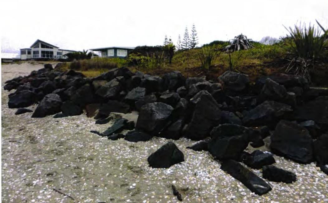
*Photo 6: Southern extent of existing structure – showing landward retreat for unprotected area*
