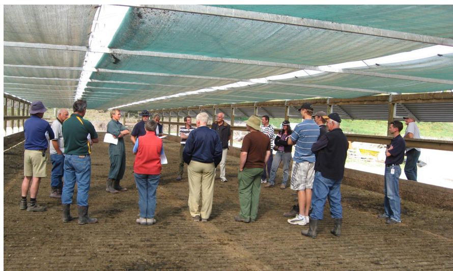
Inside the Herd Home animal shelter. Note the slatted floor over the effluent bunker. Shade cloth keeps the herd cool in summer and is drawn back to keep cows warm in winter under the clear roof.
