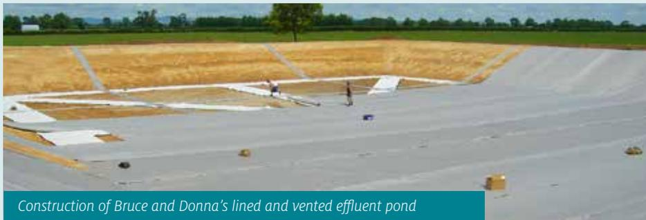
Construction of Bruce and Donna's lined and vented effluent pond
