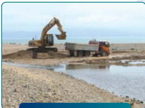
Flood protection work is underway on the Thames Coast.
